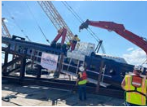
Figure 8: Pipe pusher installed on marine barge prior to pipe pull-back operations
