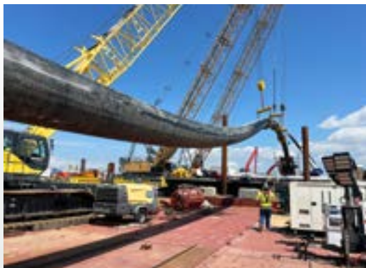
Figure 7: HDPE Pipe suspended above the marine barge during pipe pullback operations
