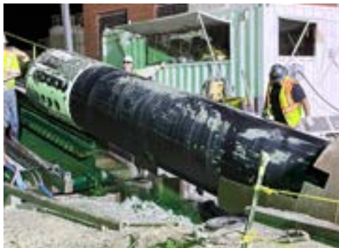
Figure 9: Pipe successfully pulled through bore back to entry pit after pipe pullback
