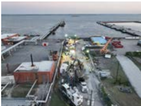
Figure 5: Aerial view of onshore entry pit and ancillary equipment and crane. View to southeast. Steel conductor casing is visible within entry pit trending southward towards shoreline
