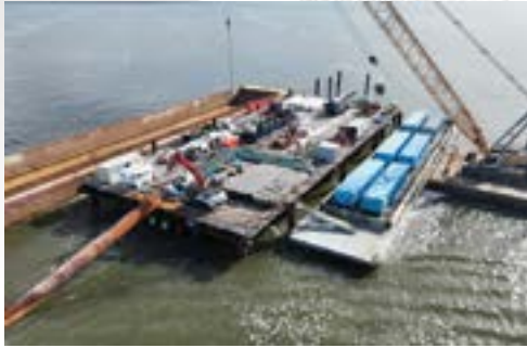
Figure 4: Aerial view of marine platform and ancillary barges and crane. View to southeast. Steel conductor pipe is visible at bottom left of image trending northward from the platform
