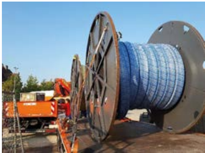
The liner folded into U-shape and coiled on reels saves transport costs thanks to its small footprint
