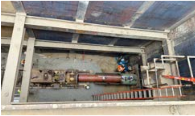
Drive lengths of over 700 feet were completed out of 14x48 FT jacking shafts averaging over 40-feet deep
