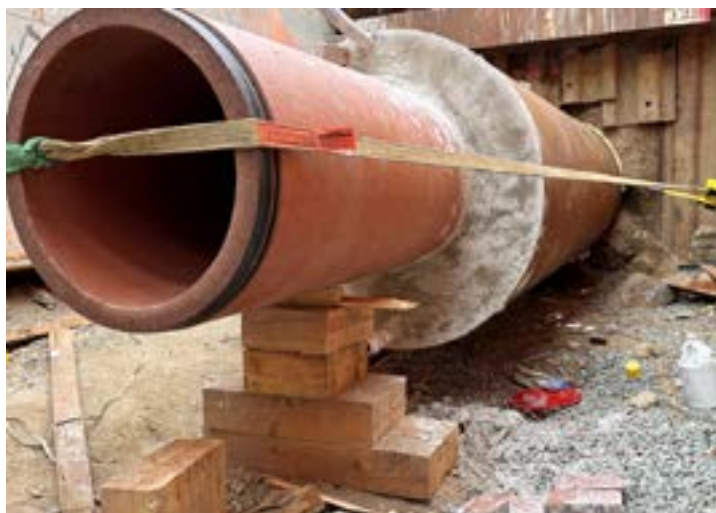
24-inch Vitrified Clay Carrier pipe within a Casing: Concrete Bulkhead/ Grout Filled Annulus
