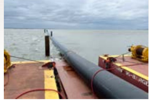
Figure 6: Aerial view of pipe-fusing barge (Figure 6A) and the fused pipe deployed out into the James River (Figure 6B)
