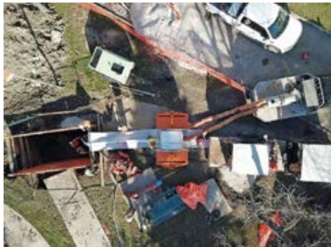
The liner folded into U-shape and coiled on reels saves transport costs thanks to its small footprint
