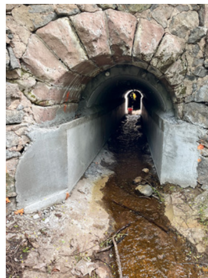
Non-circular geometry makes traditional sliplining impractical
