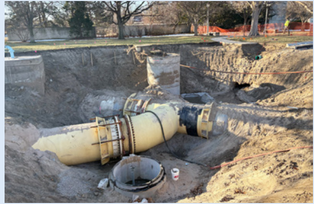
The 90-degree turn through a tee that led to the newly constructed section of pipeline towards the retrieval point
