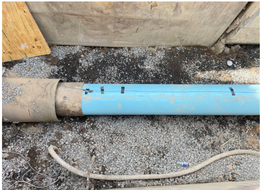
18-inch Fusible PVC pipe insertion into existing 24-inch ductile iron pipe
