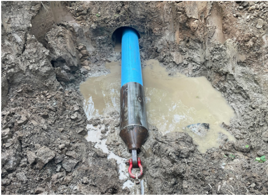
18-inch Fusible PVC slipline completed in existing 30-inch cast iron pipe
