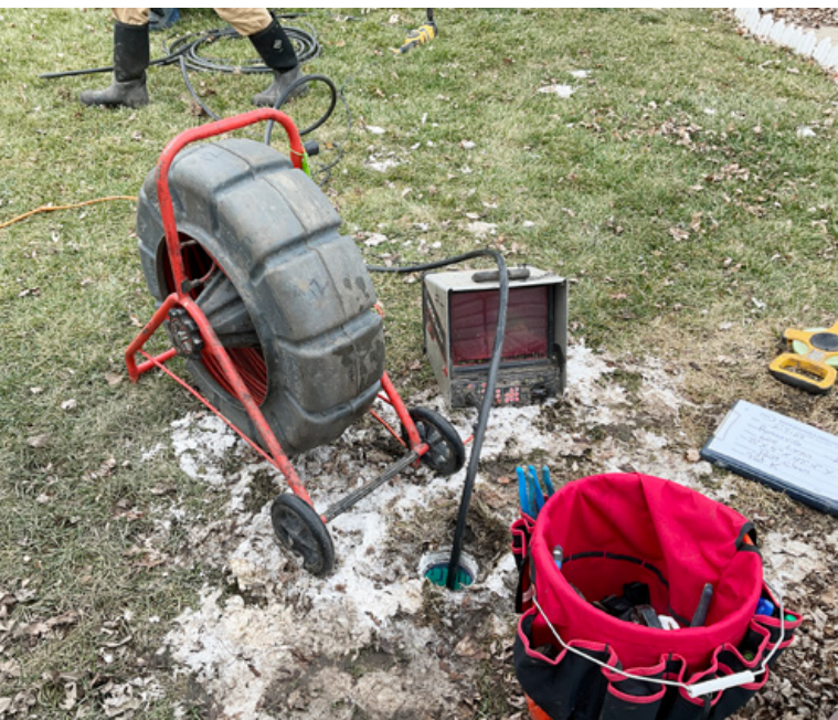
Figure 7. Push Camera setup – allows PPI to follow liner as it is extended into lateral during installation – crew uses to ensure liner is sticking to host pipe correctly prior to beginning curing
