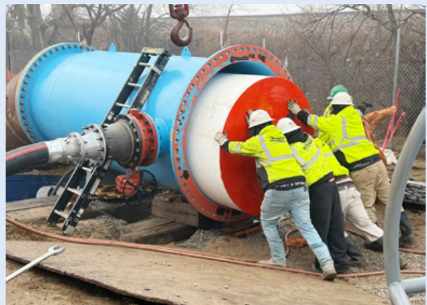
An external pump was used to launch the pig into the pipeline until the point that it was propelled by the system water flow
