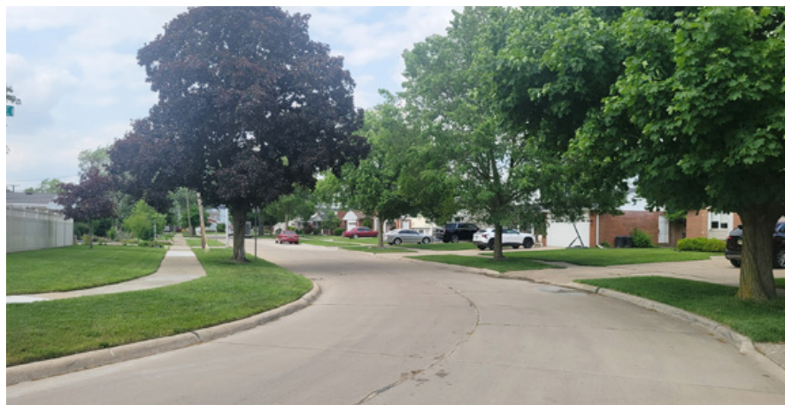
The Riverview neighborhood, built in the 70s, needs expanded sewer overflow service to eliminate basement flooding
