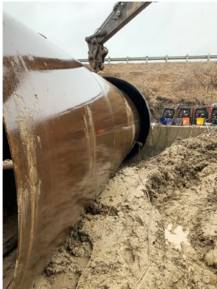
Installing Steel Casing Liner Pipe
