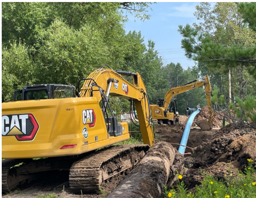
Geislinger & Sons completing slipline installation at entry pit
