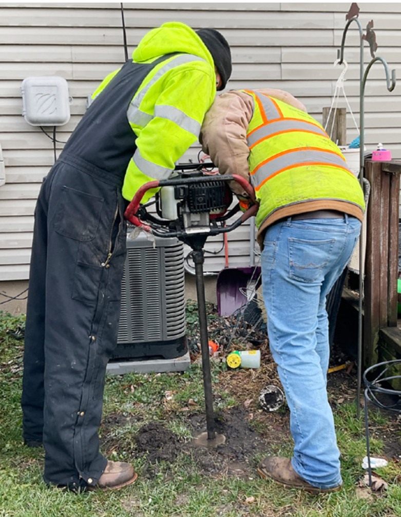
Figure 4. Coring of existing service lateral as part of Vac-A-Tee installation process
