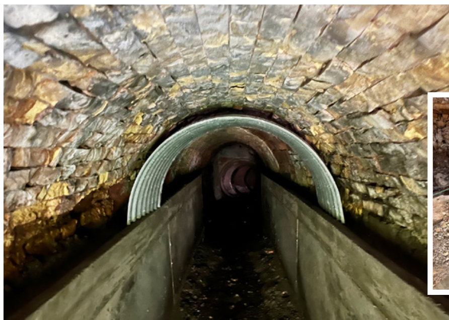
Custom-fabricated half-round liners create a snug fit with minimal annular space
