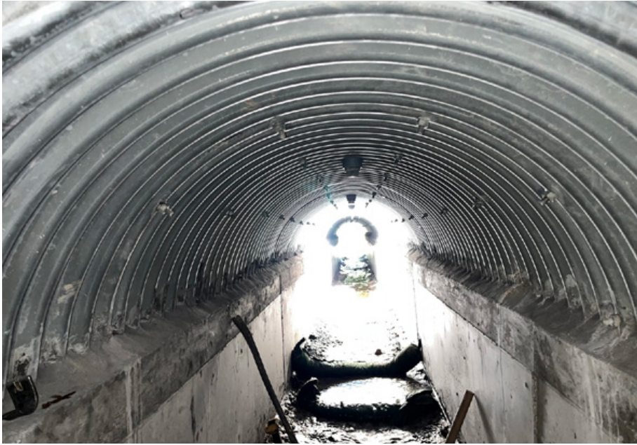
Non-circular geometry makes traditional sliplining impractical
