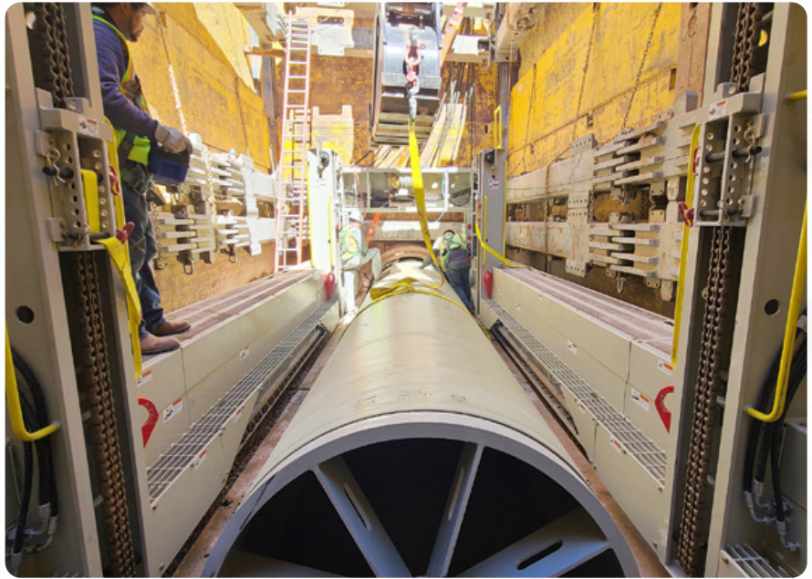
Figure 2: Rehabilitation crews sliplining FRP with an Akkerman SLS-100 frame.
