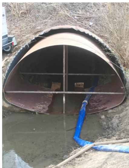
Installed InfraSteel Liner Pipe
