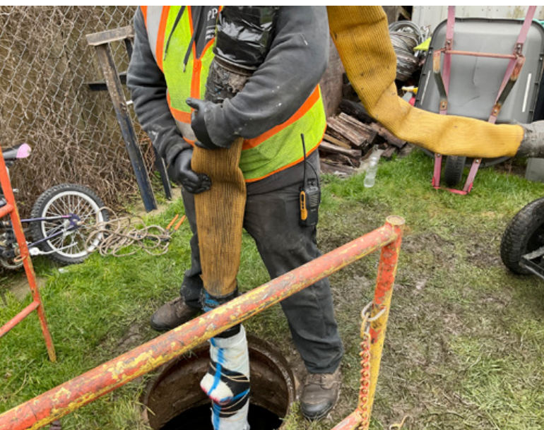
Figure 6. Feeding of Lateral Tee-Liner into manhole – Liner installation process
