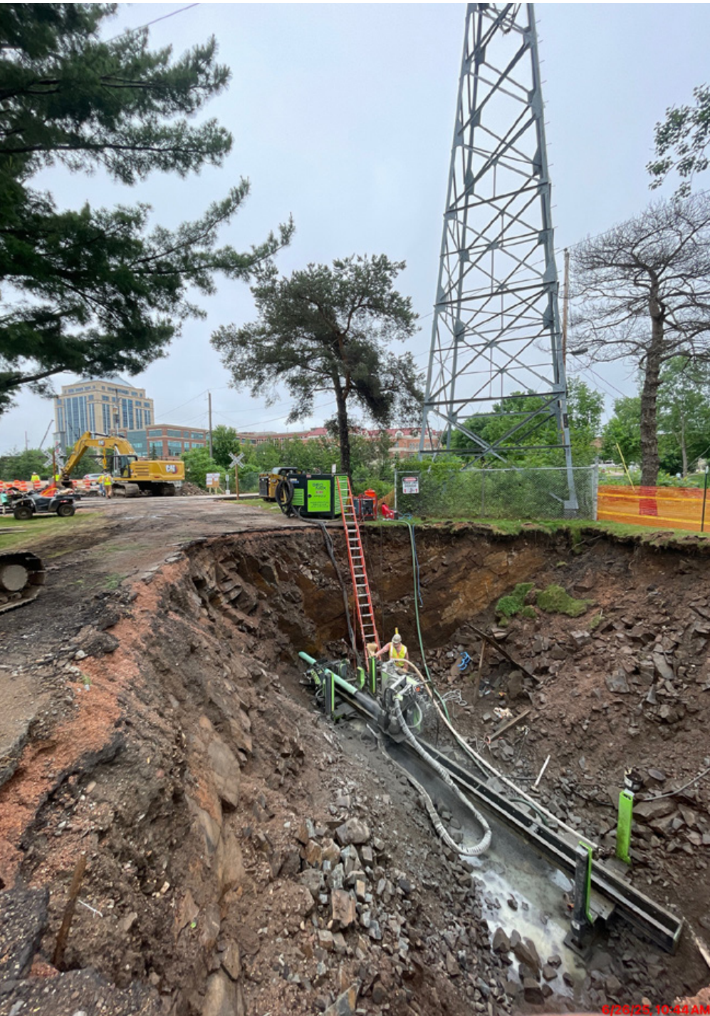
EBI Drilling utilizes their GEONEX HZR220 to install 100 feet of 6-inch steel casing below railroad tracks in less than 8 hours. Before an additional 160 feet the next day
