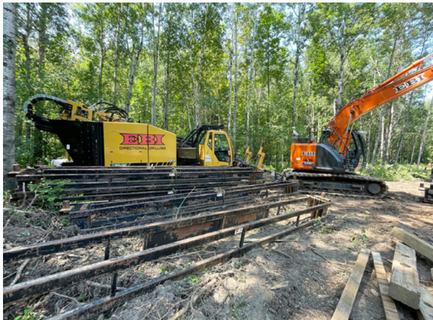
EBI Drilling completed long slipline pulls with directional drill rig
