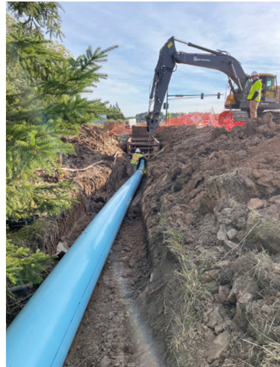
Minger Construction completing slipline installation with excavator
