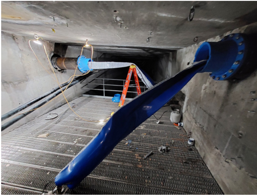
Space was restricted in the access chambers beneath the bridge
