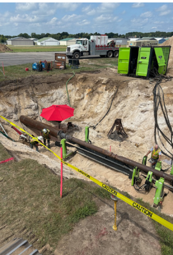
EBI utilizes their GEONEX HZR610 drill machine and power pack, complete with front extension frame to install 40-foot lengths of casing through sand and cobbles in July 2024
