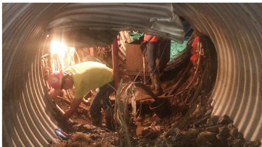
Confined space entry inspection performed before lining
