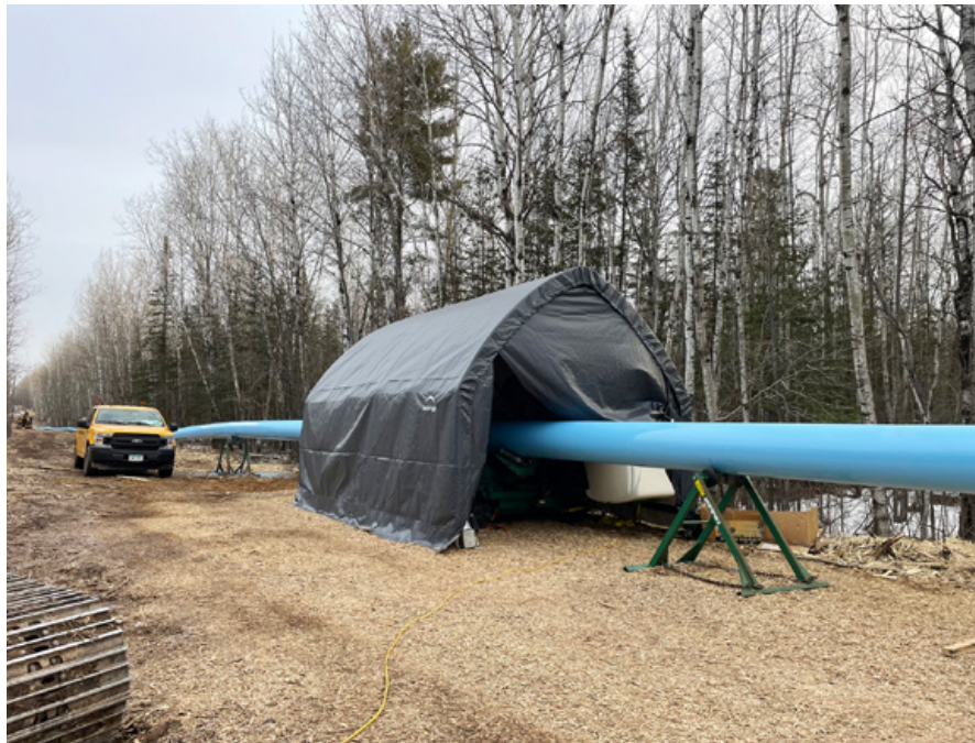
Winter pipe fusion work by Core & Main occurred in a heated structure
