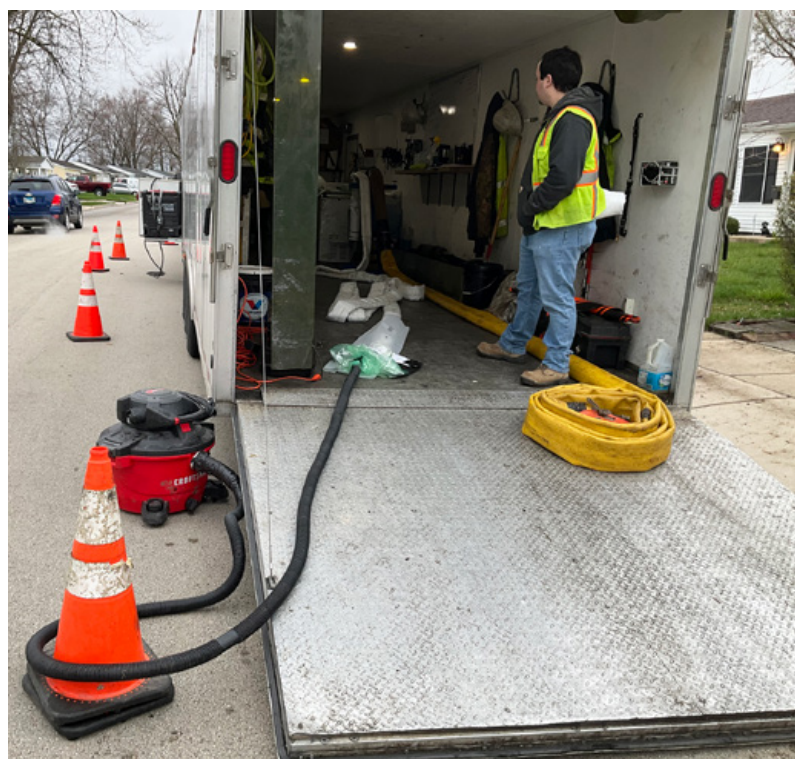
Figure 3. Use of a shop-vac to pull resin through the entire length of the T-Liner™ as part of resin saturation
