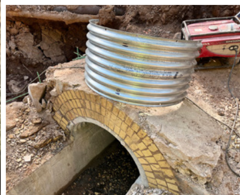
Custom-fabricated half-round liners create a snug fit with minimal annular space
