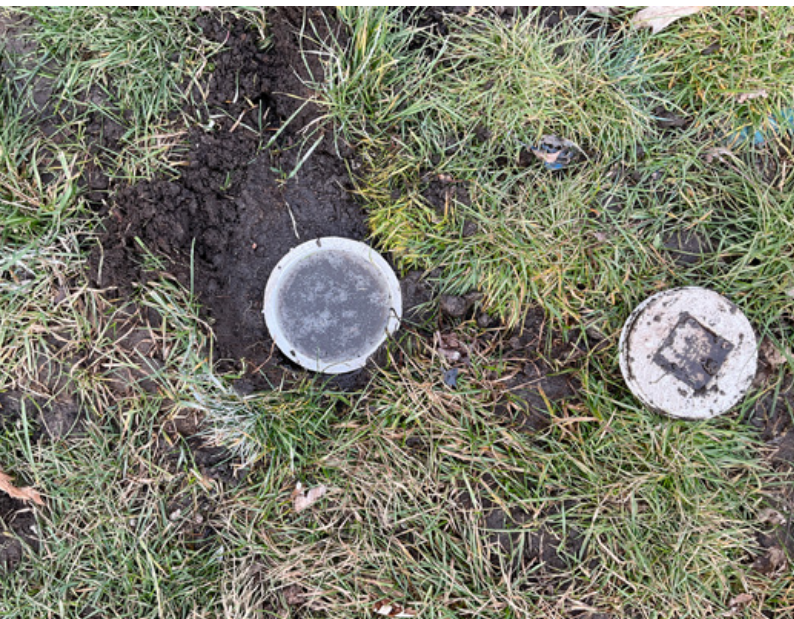
Figure 5. Hydrostatic Test performed on installed Vac-A-Tee to ensure the cleanout is properly sealed from any potential infiltration
