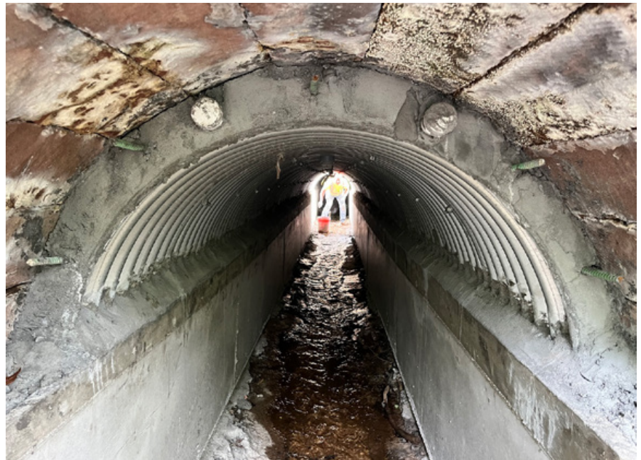
Arch-shaped culverts present unique obstacles for engineers
