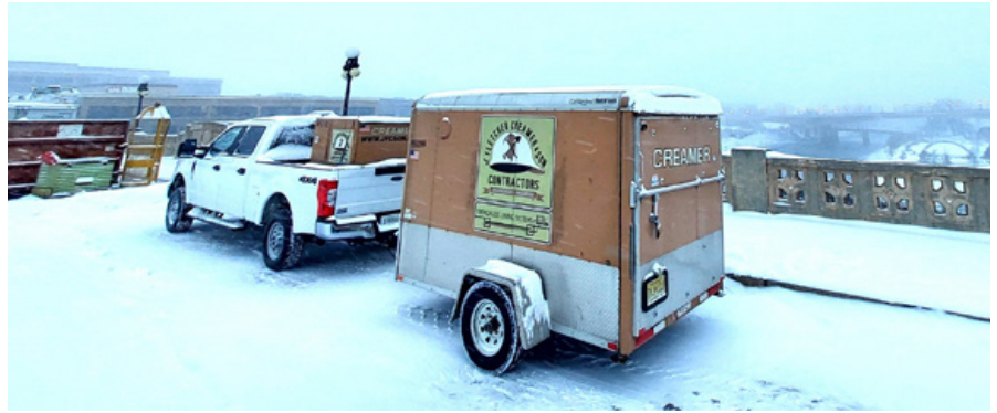
Access to the watermain limited to manholes located on the bridge deck
