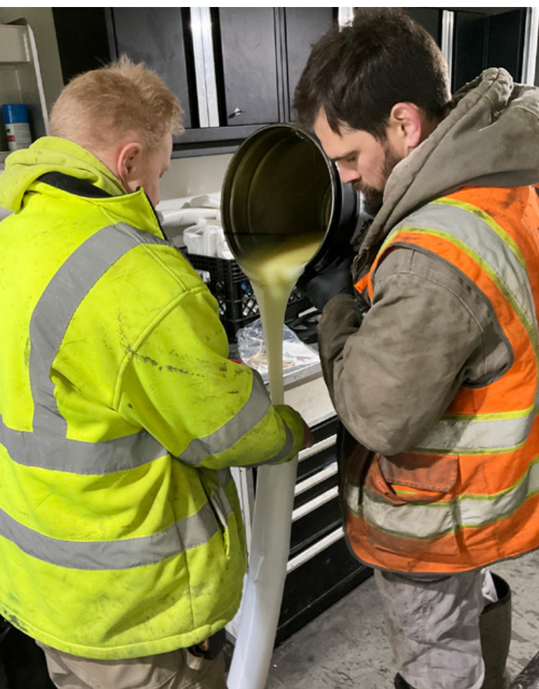
Figure 2. PPI Crew prepares the lateral liner w/ resin saturation
