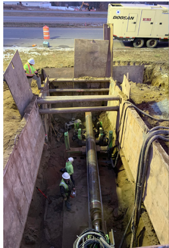
From the Launch Pit: EBI's operator uses the GEONEX wireless remote control to operate their HZR610 Drill machine for a 320-foot installation below the highway
