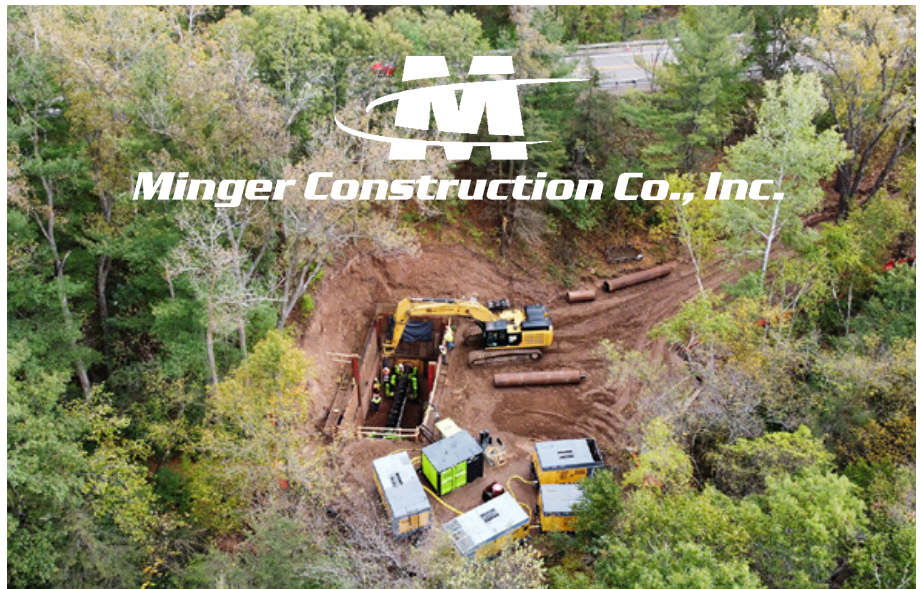
Minger Construction completing slipline installation with excavator
