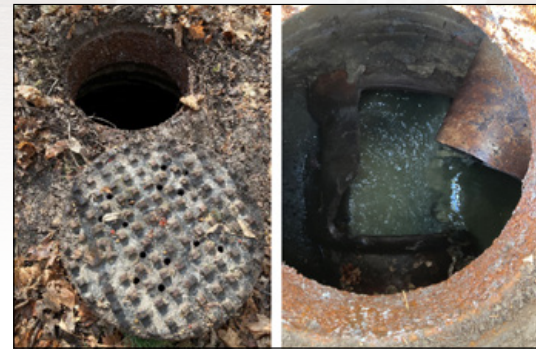
Figure 6: Existing Manhole MH-5294
