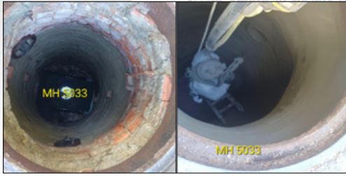
Figure 18: Manhole 5033 Pre-lining and cementitious lining application
