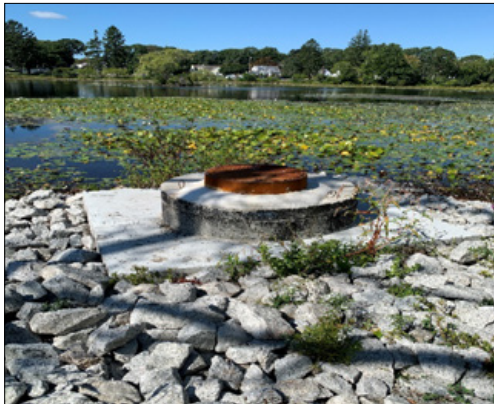
Figure 20: Rehabilitated manhole MH-5035
