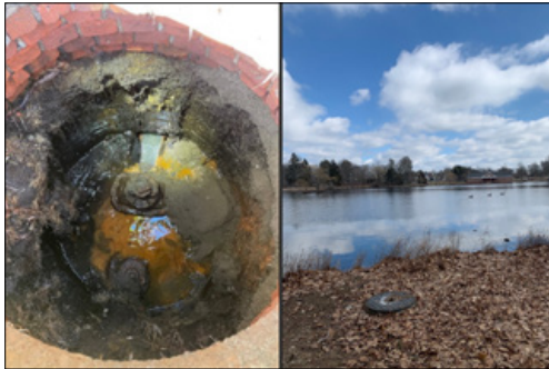
Figure 19: Existing manhole MH-5089
