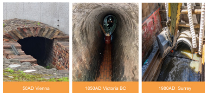
The function and design of pipes has changed very little in the last 2000 years
