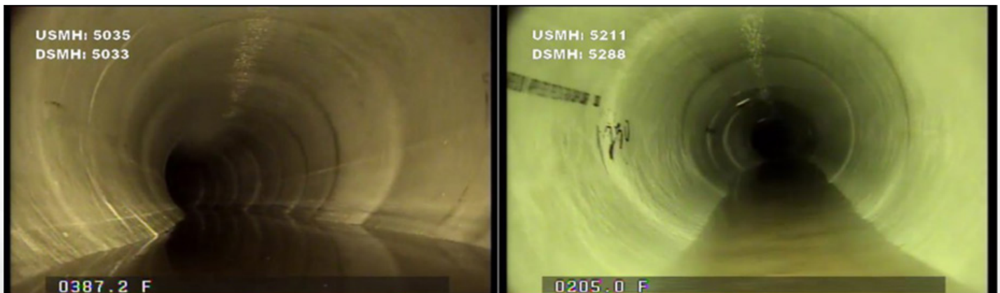
Figure 21: Installed liner along 36-inch GSC at the horizontal bend downstream of manhole MH-5035 (left photo) and installed liner along 18-inch lateral sewer (right photo)
