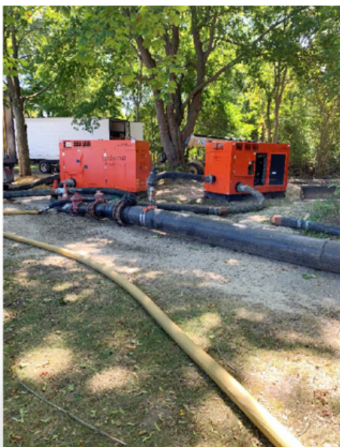
Figure 13: Bypass Pumps at Upstream GSC Manhole
