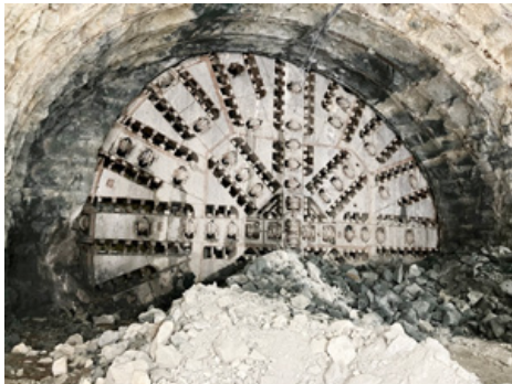
The 13.67 m (44.87 feet) diameter Robbins Slurry machine broke through this spring in Hiroshima, Japan
