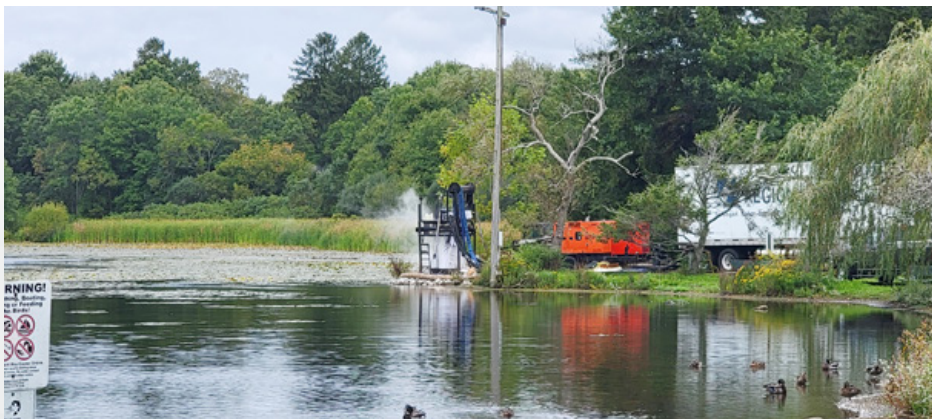
Figure 17: CIPP Installation at MH-5035
