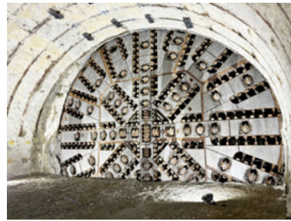
The mega-sized machine for the Obayashi-Taisei-Kosei joint venture bored the Hiroshima Expressway Line 5 tunnel
