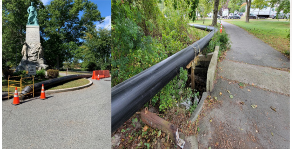
Figure 14: Bypass Discharge at MH-5034 and Brook Crossing
