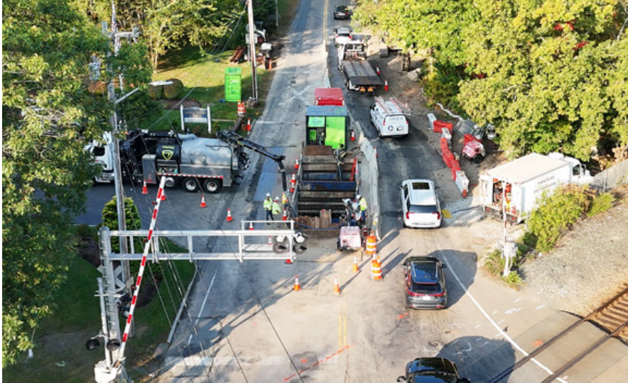
The launch pit was located in a narrow strip of the roadway between single lane opposing traffic
