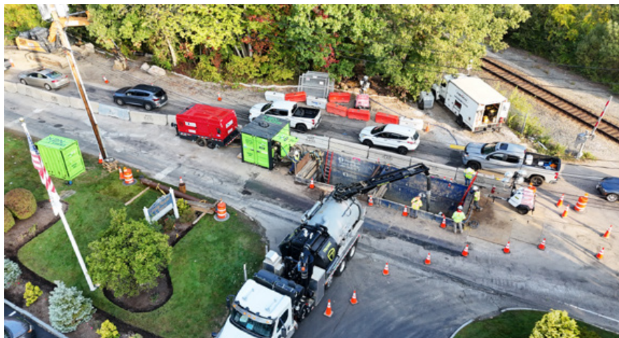
A new 12-inch gas main was installed below a high speed MBTA track
