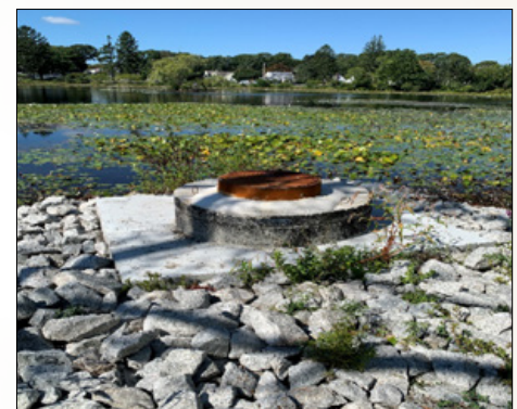
Figure 20: Rehabilitated manhole MH-5035
