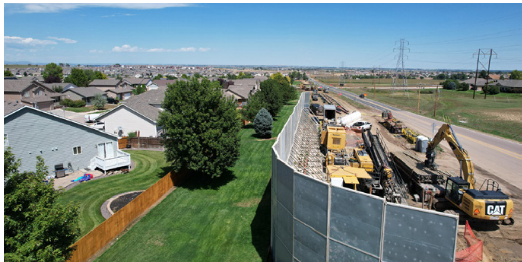
Freestanding panels provide noise mitigation for HDD project near a usually quiet neighborhood
