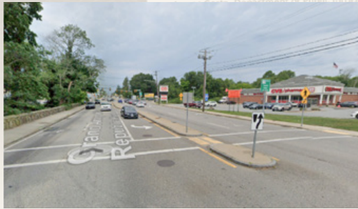
Figure 12: Kempton Street looking west at upstream manhole on Grape Street Collector located in the median
