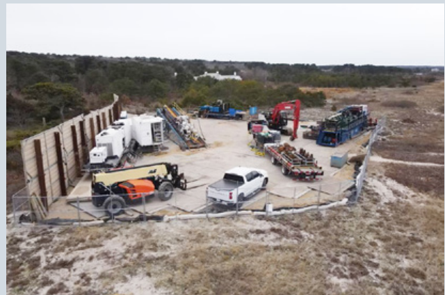
Barriers effectively reduced noise from all drilling and equipment staging areas
