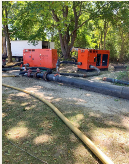
Figure 13: Bypass Pumps at Upstream GSC Manhole
