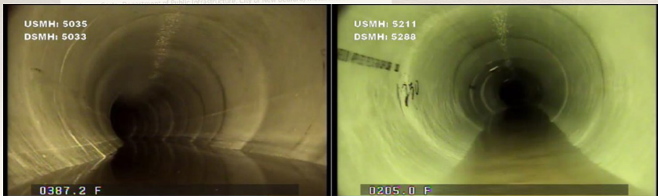
Figure 21: Installed liner along 36-inch GSC at the horizontal bend downstream of manhole MH-5035 (left photo) and installed liner along 18-inch lateral sewer (right photo)
