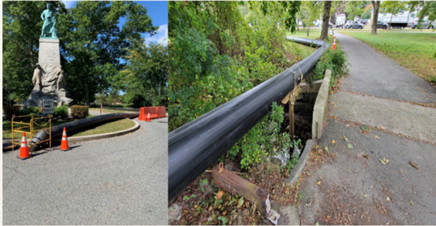
Figure 14: Bypass Discharge at MH-5034 and Brook Crossing
