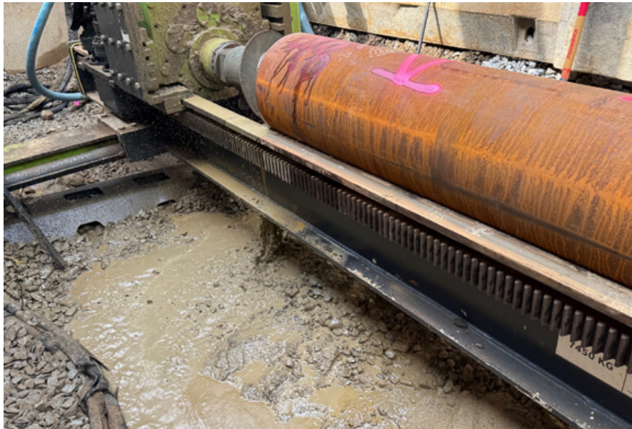
System bored efficiently through solid granite, cobbles, boulders, clays and mixed face conditions with an astounding success rate
