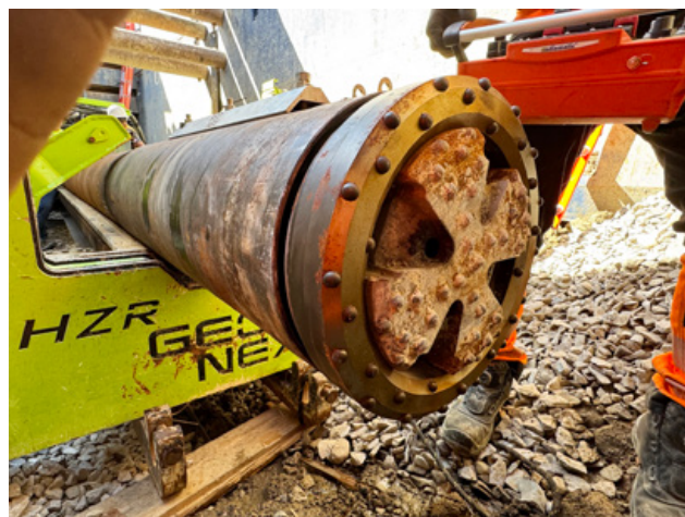
Down Hole Tooling ready to begin
