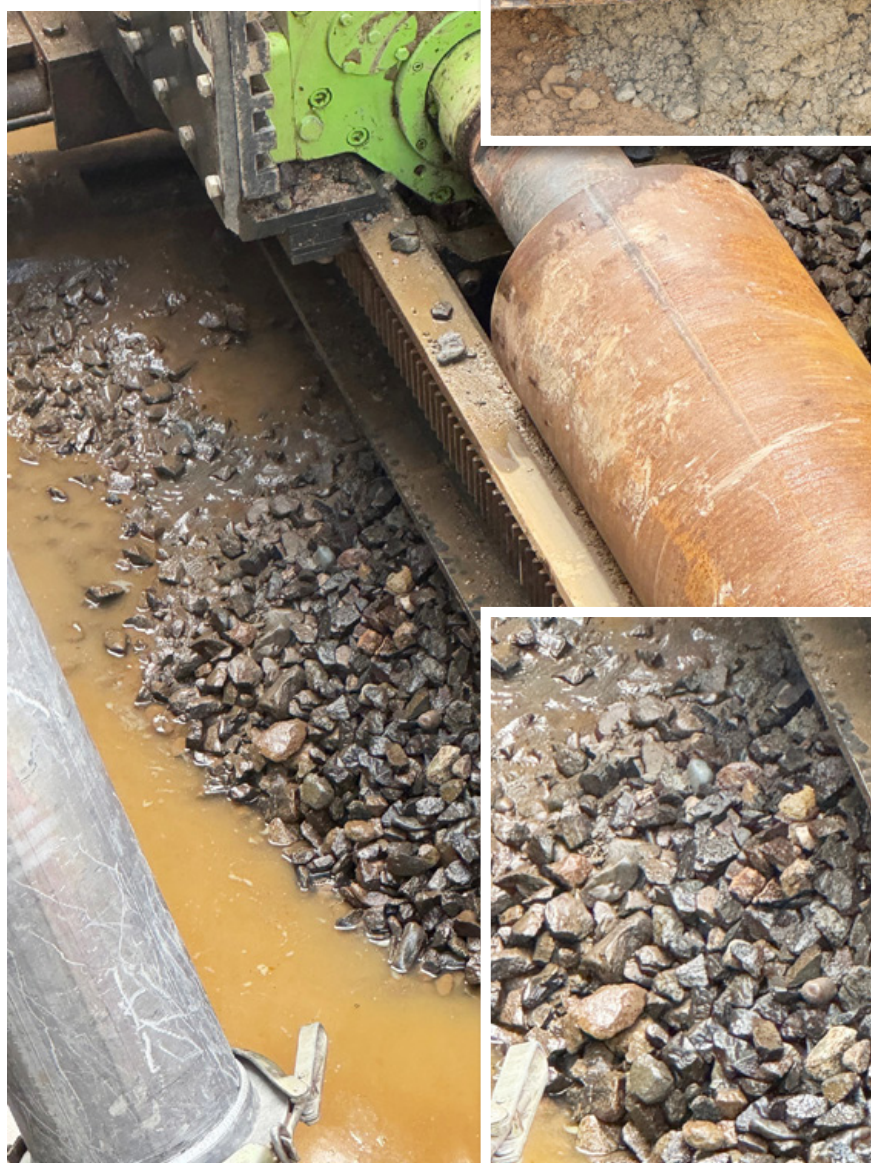
Mixed face conditions were encountered throughout the installation
