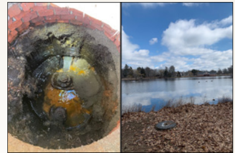
Figure 19: Existing manhole MH-5089
