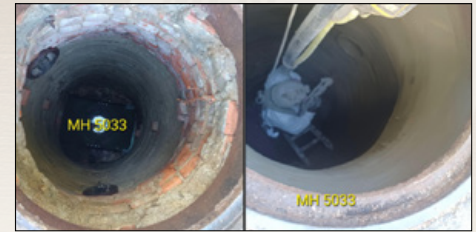
Figure 18: Manhole 5033 Pre-lining and cementitious lining application
