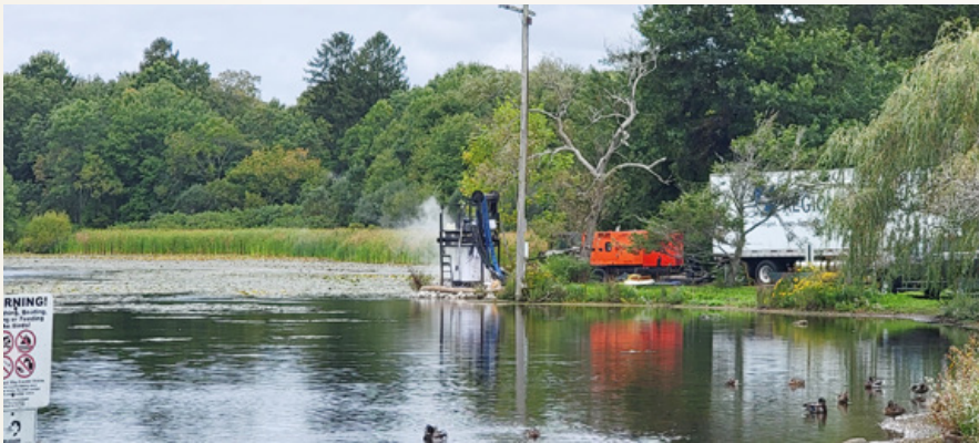
Figure 17: CIPP Installation at MH-5035
