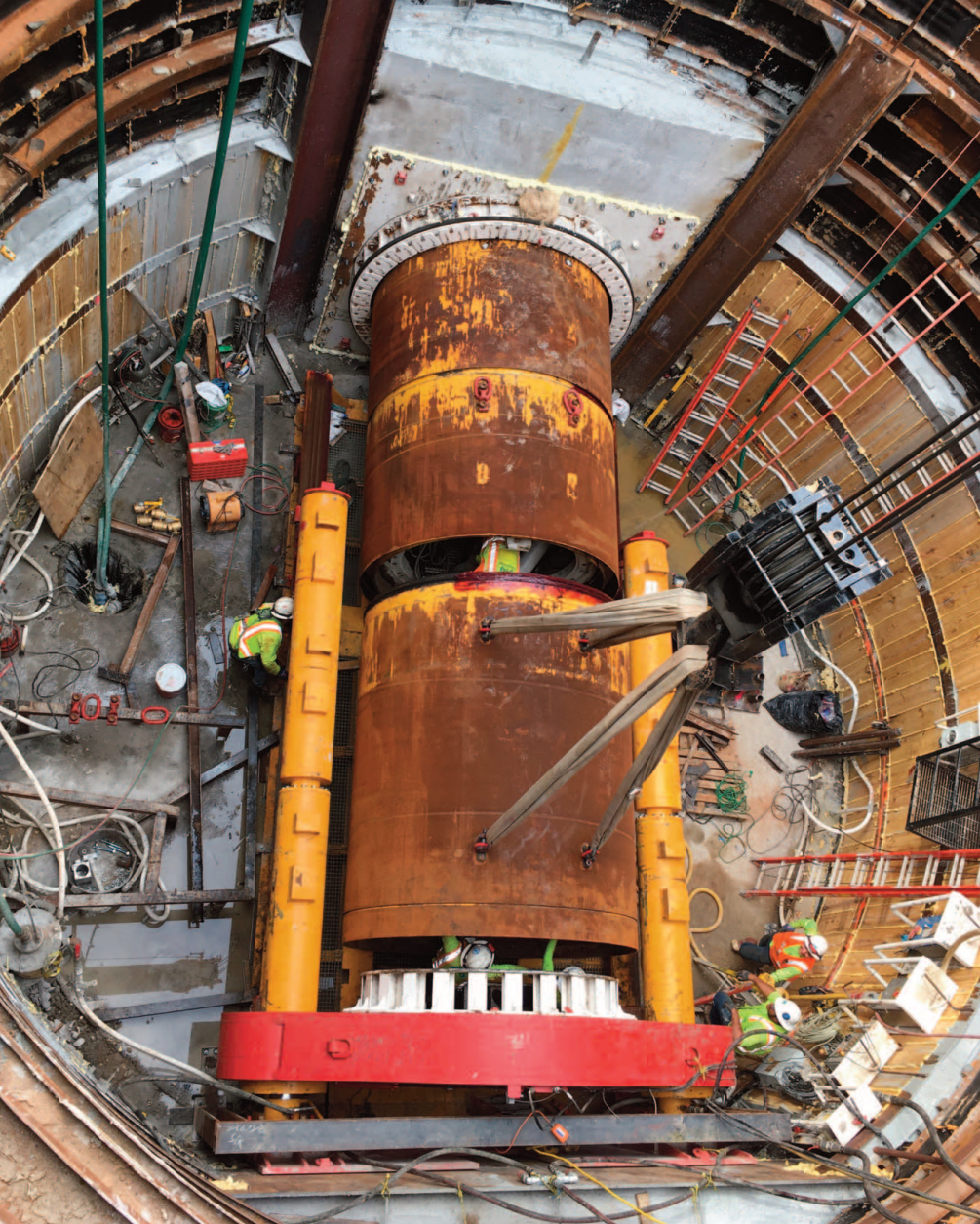
Figure 3. Herrenknecht AVN 2000AB microtunneling boring machine in use along with interlocking steel casing
