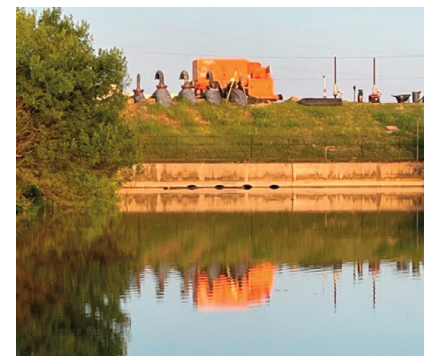
Figure 6. Discharge Outfall Access Surcharged During Flood (Source: Stephens and Peterie 2025)
