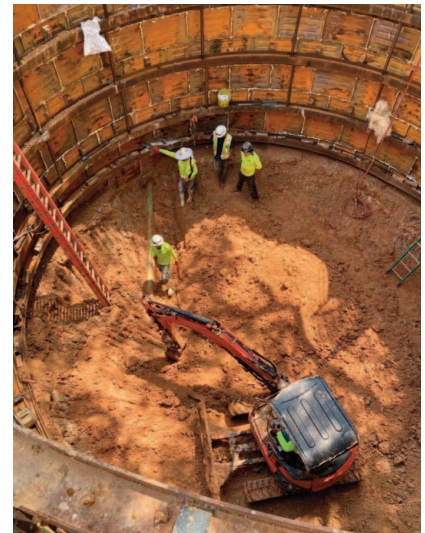
Figure 4: Newer idle 6-inch HDD pipeline found at the White Oak Bayou launching shaft
