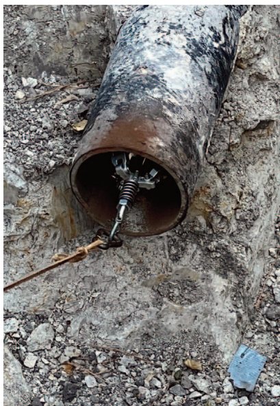
Figure 5: Wireline survey used to map exact location of 6-inch steel pipeline discovered during construction
