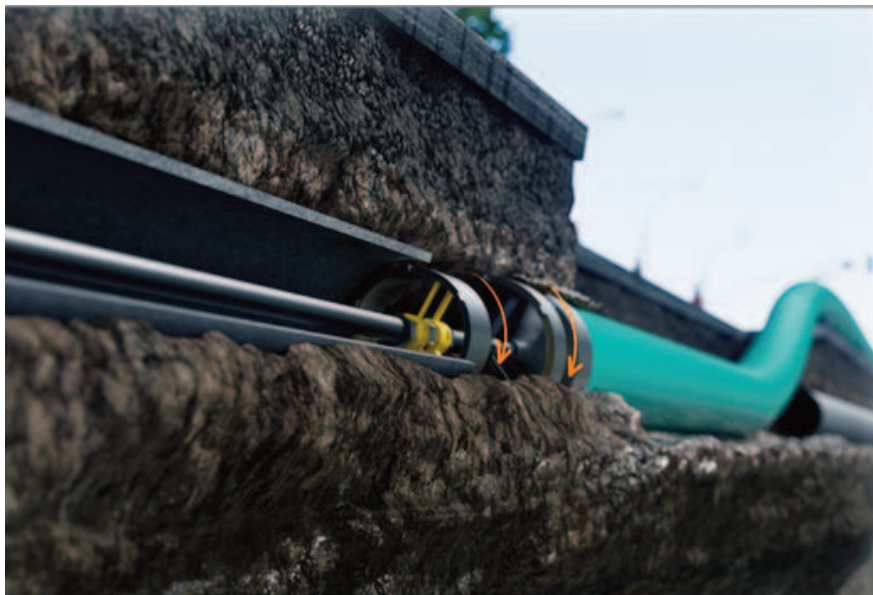
Figure 1. The CTPS process grinds the existing host pipe while simultaneously pulling in new pipe
