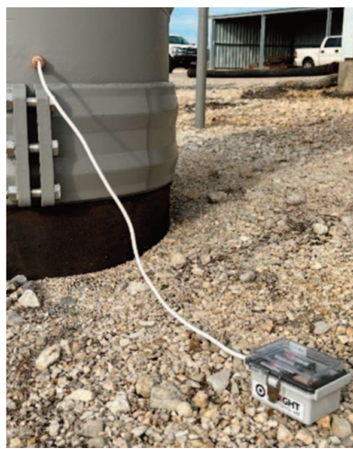
Figure 4. Tracking Unit Along Alignment
