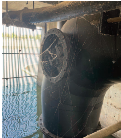
Figures 3 (left) and 4 (right). Access at Vents at Levee Crest (left) and Inside Pump House on Pump Intakes (right) (Source: Stephens and Peterie 2025)
