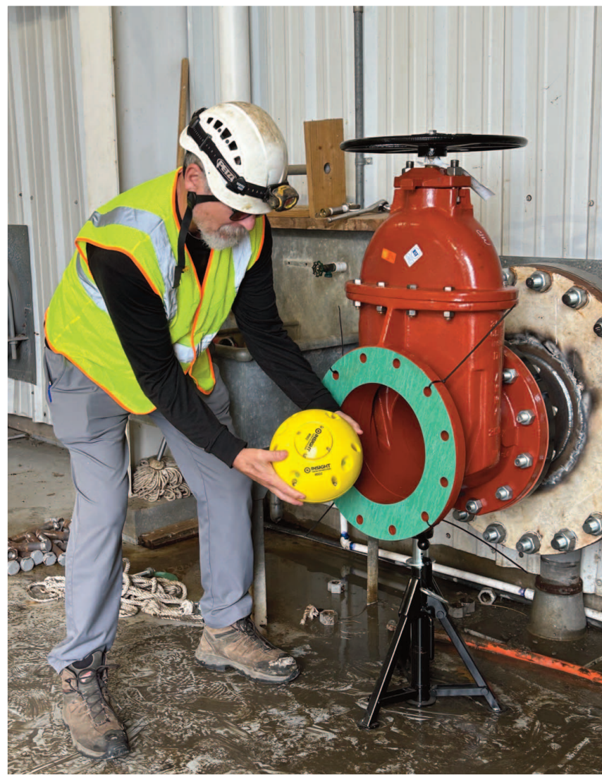
Figure 3. Insertion of Ball Through Modified Flange at LNRA Pump Station
