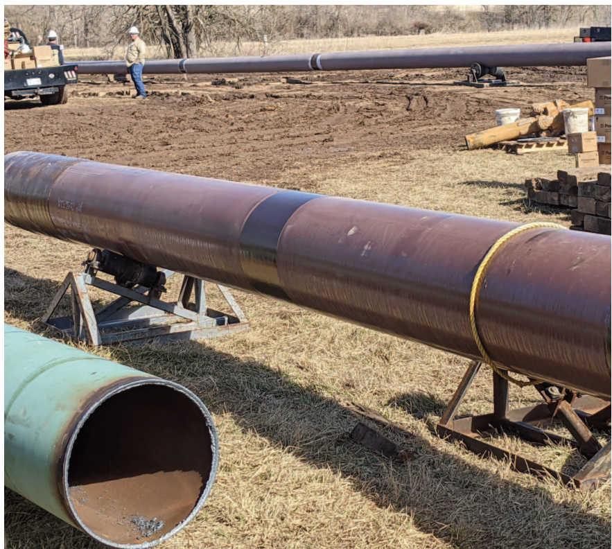
Visual comparison of three coating sections post-HDD: 4-layer Bore-Wrap (front), epoxy ARO (middle), and 2-layer Bore-Wrap (rear)
