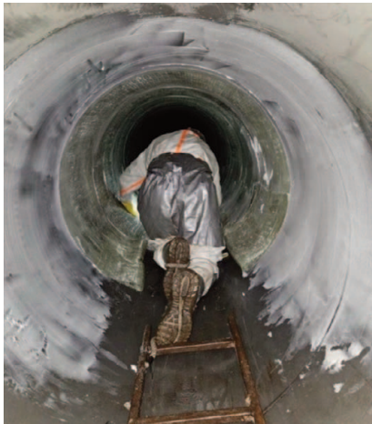
Figures 10 (left) and 11 (right). Sloped Pipeline Access Challenges (Source: Stephens and Peterie 2025)
