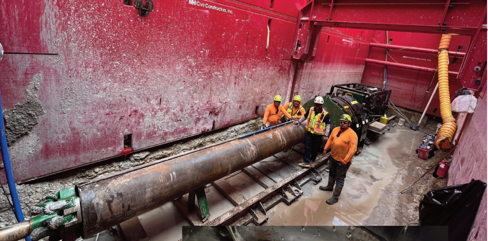
Figure 3: Guided auger boring offers production and accuracy in competent, predictable soils
