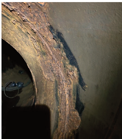
Figures 7 (left) and 8 (right). Coating Prior to Surface Preparation (left) and Coating Being Removed (right) (Source: Stephens and Peterie 2025)
