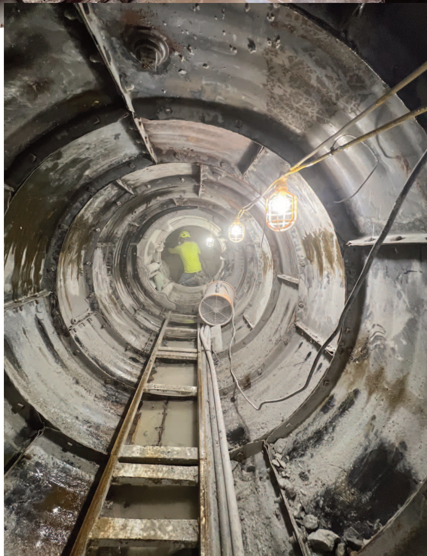
Figure 4: Hand tunneling provides flexibility and face control in variable or unstable formations
