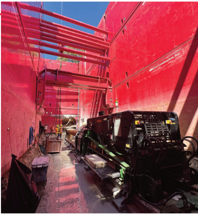
Figures 5 and 6: Deep shafts required engineered trench boxes/shoring, and robust safety protocols
