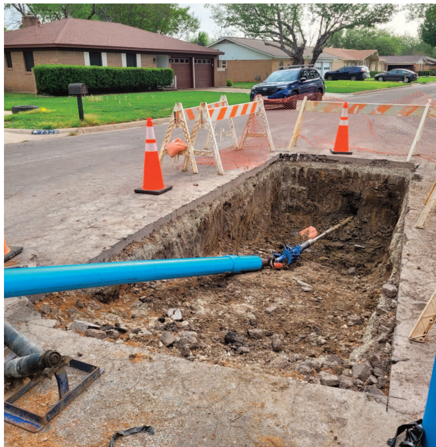
The reamer and pulling head are attached to a short length of Certa-Lok
