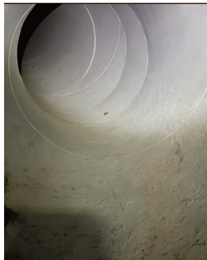
Figure 9. Surface Preparation to Near White Metal Finish (Source: Stephens and Peterie 2025)
