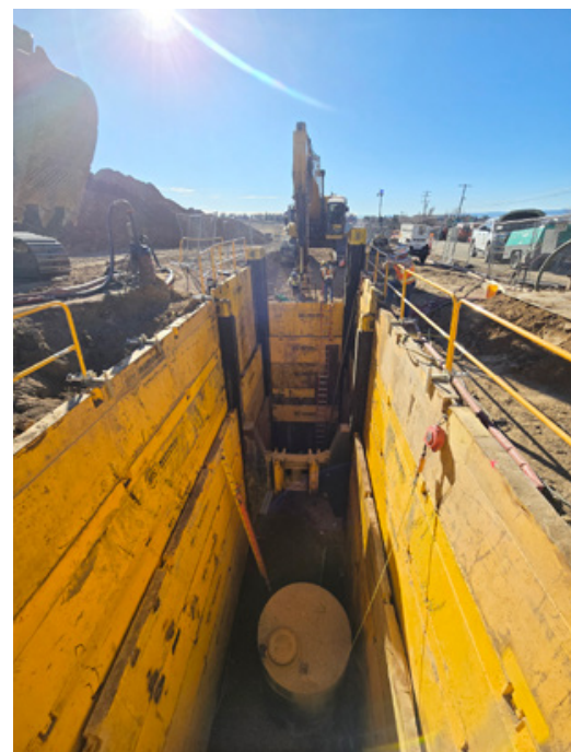
Shaft 300, Manhole has been installed the crew is working to remove the slide rail system and backfill the shaft under tight tolerances
