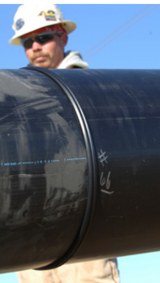
Heat fusing HDPE pipe sections provides a leak-free joint plus heightened security and protection from seismic events
