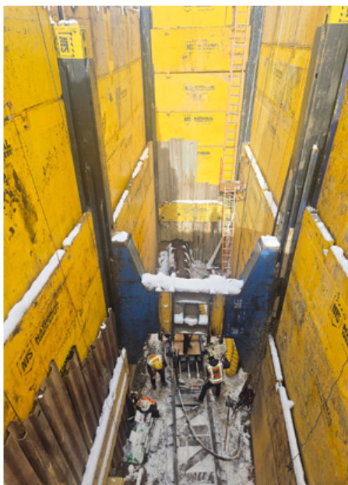
Shaft 300, Preparing shaft for the start of hand mine tunneling operations
