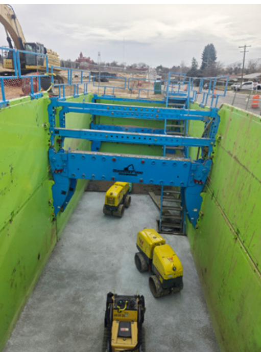
Shaft 100, Carrier pipe installed and preparing shaft for installation of manhole
