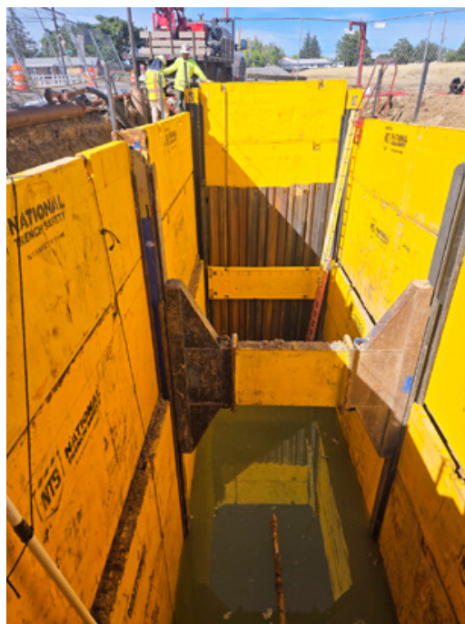
Shaft 200 Slide rail with ground water present after generator cables were stolen over the weekend shutting off the dewatering system on site
