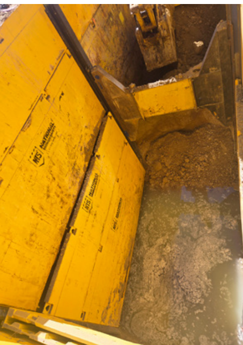
Shaft 200 slide rail installation with ground water present in shaft bottom
