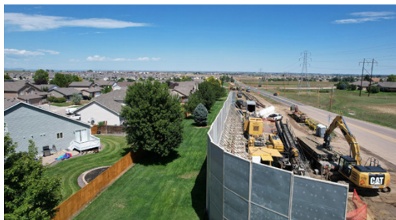
Freestanding panels provide noise mitigation for HDD project near a usually quiet neighborhood
