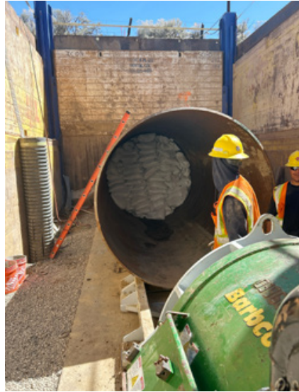
Sandbag Plug in the lead casing
