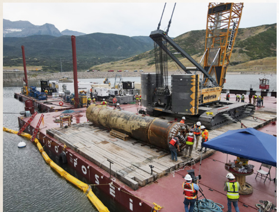
Figure 6: Wet recovery of MTBM
