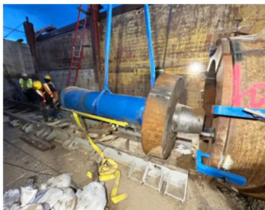
The casing had to be split in order to extract the hammer
