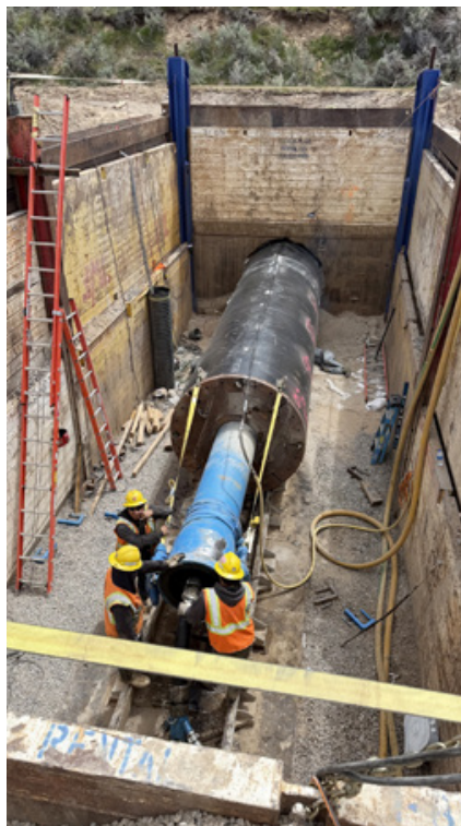
Accomplished the largest diameter pipe ram in the state of Utah
