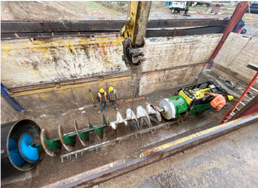
Cleaning out the casing
