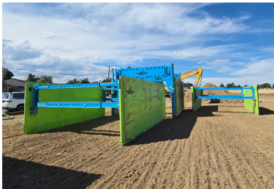
GroundWorks shoring system prior to installation within Shaft 100
