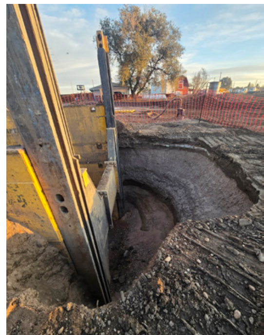
Shaft 200 loss of ground due to surface water flows over the weekend
