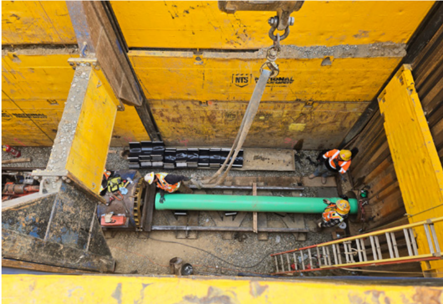
Shaft 200, Installing carrier pipe from shaft 200 towards shaft 100
