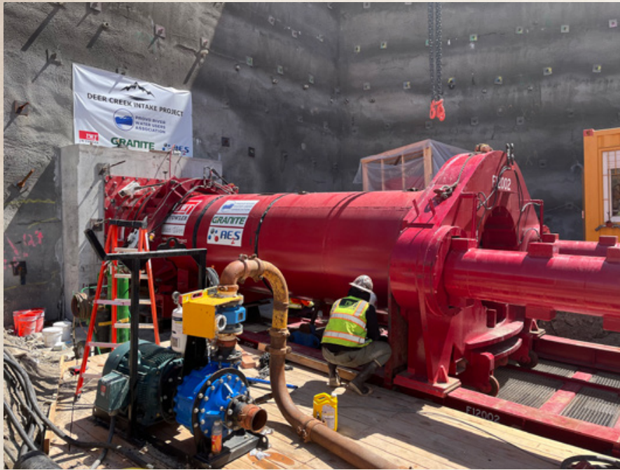
Figure 4: MTBM launch portal
