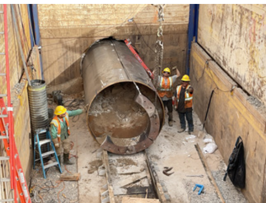
Material settlement packed against the hammer face
