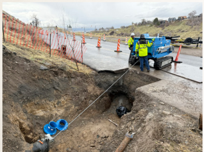
Figure 6: Pulling liner into pipe using 10-ton pulling winch
