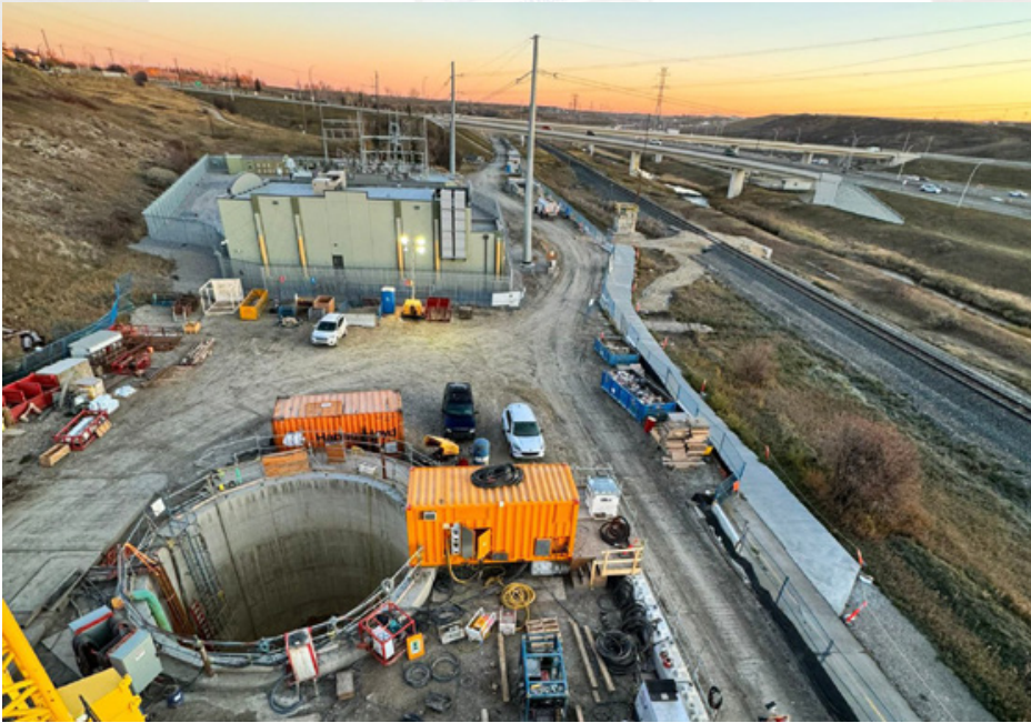
Figure 2. View of main tunnel launch shaft looking north (Note: ENMAX substation, CPKC tracks, and Nose Creek shown)
