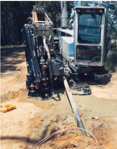
Bare conductor was installed with bentonite, providing stability and electrical connection
