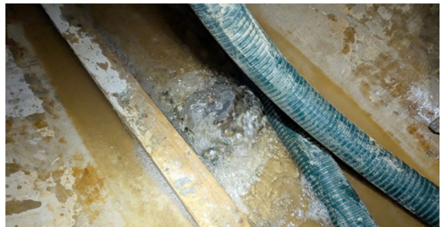
Figure 11. Infiltration during Sliplining and Annular Dewatering into Inserted FRPM Pipe
