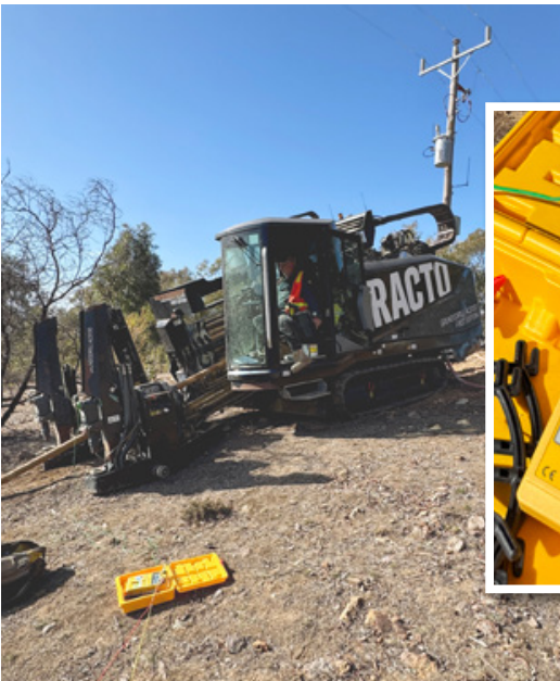
Resistivity measurements were taken as the installation progressed
