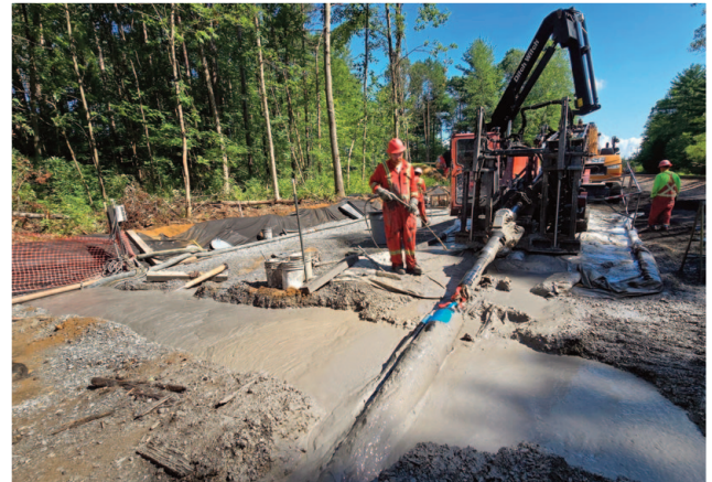
In gas infrastructure construction, the ground is rarely cooperative
