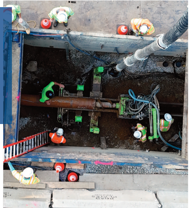
Down Hole Tooling ready to begin
