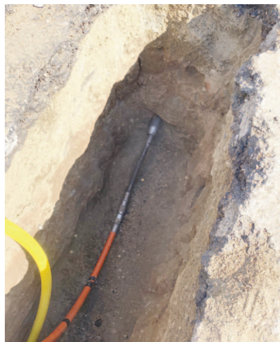
Piercing tools are a staple in the gas industry for service line installations because they are trenchless and accurate
