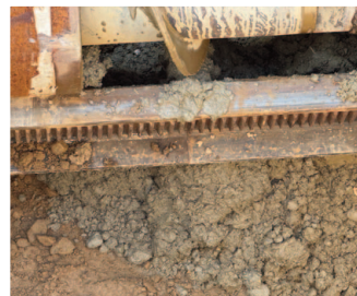
Mixed face conditions were encountered throughout the installation
