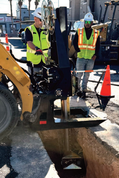
LEFT: Existing service lines are replaced along their original alignment without continuous open-cut excavation. RIGHT: Typical service-splitting equipment.
