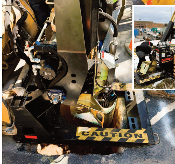
LEFT: Existing service lines are replaced along their original alignment without continuous open-cut excavation. RIGHT: Typical service-splitting equipment.
