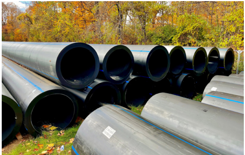
The Waterbury water transmission line project used 42-inch SDR11 PE4710 HDPE IPS pipe manufactured by JM Eagle that has a wall thickness of 3.82 inches and is rated for 200 PSI working pressure
