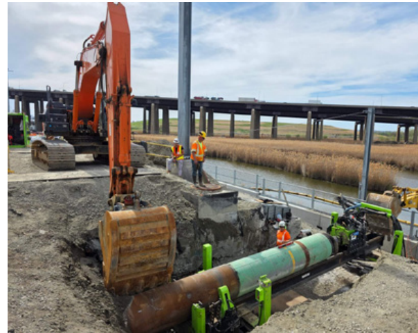
HHB utilizes a pneumatic hammer at rock face while simultaneously advancing the casing
