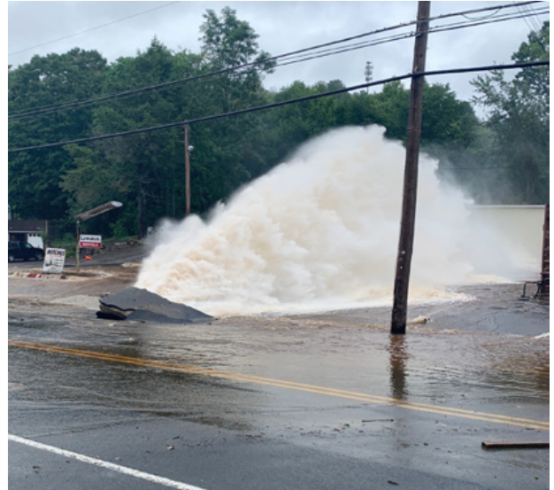
This geyser caused by one of the breaks in Waterbury's 200 psi potable water transmission lines launched sizable buried rocks into the air, damaging a nearby garage
