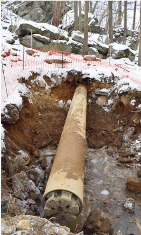
The 24-inch starter casing (ring bit removed) advanced through the centralizing system and exited within the project's required line and grade tolerances
