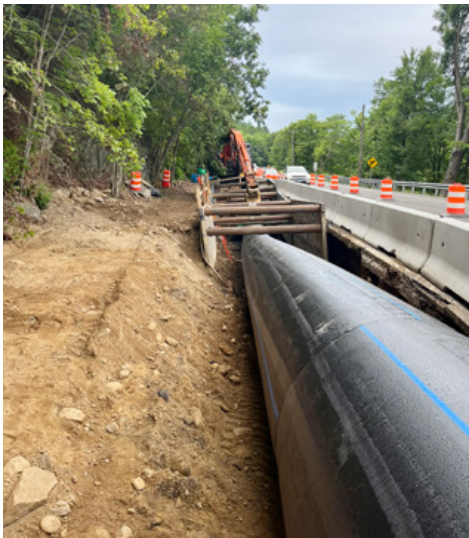
The Waterbury water transmission line project used 42-inch SDR11 PE4710 HDPE IPS pipe manufactured by JM Eagle that has a wall thickness of 3.82 inches and is rated for 200 PSI working pressure
