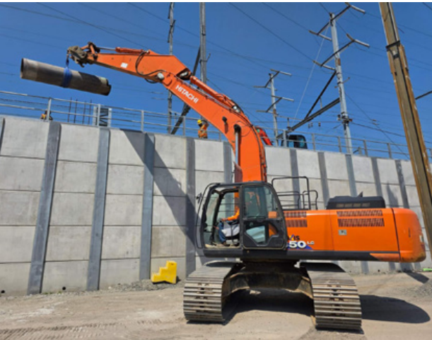
HHB utilizes a pneumatic hammer at rock face while simultaneously advancing the casing
