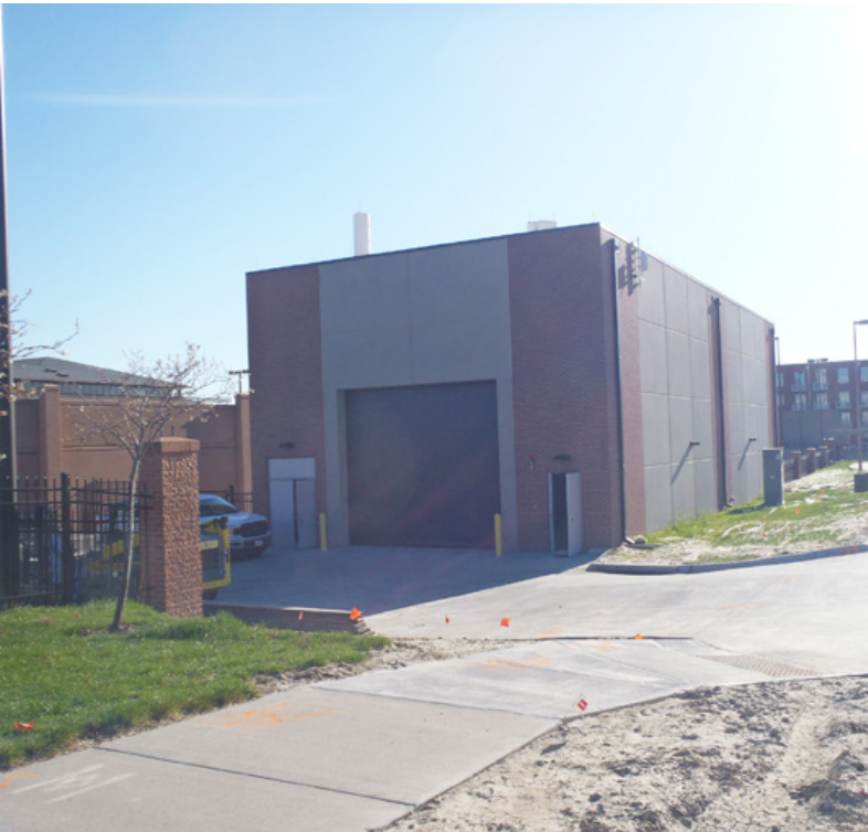
Figure 6. New Grit Facility
