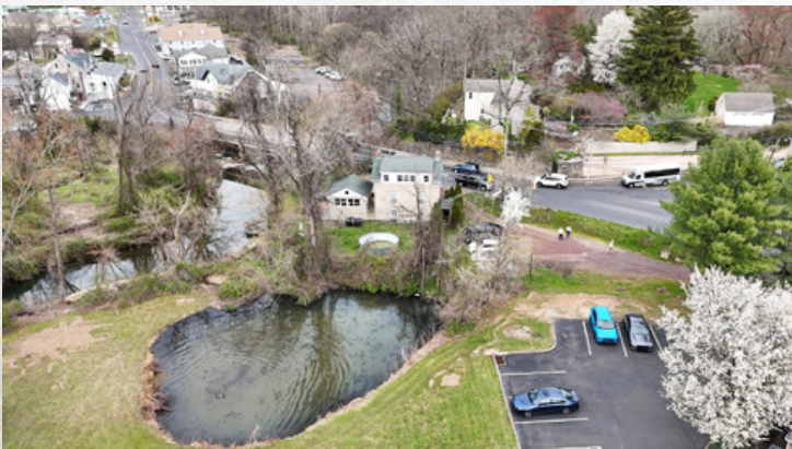
The bore alignment paralleled Mill Creek within a constrained easement, limiting construction access that eliminated conventional open-cut installation
