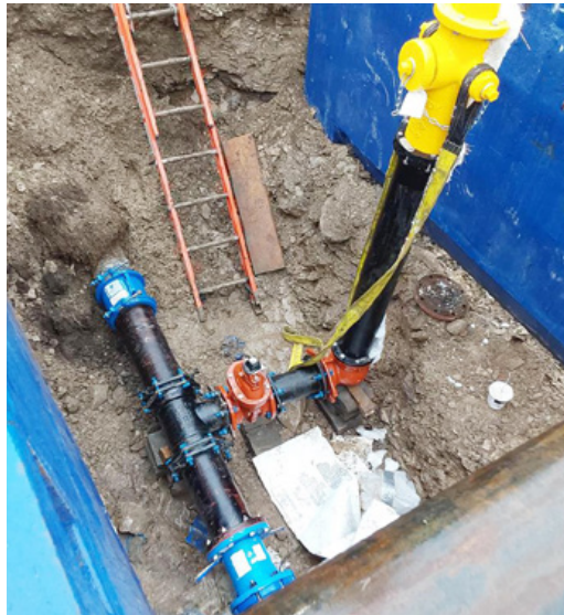
New fire hydrant, isolation valve and valve box installed
