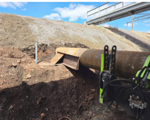
Shown above, some of the site constraints of the Portal North Bridge Project. NJ based trenchless contractor Kmetz Inc utilized their HHB equipment on this project and now deploys it on nearly every project where rock is anticipated
