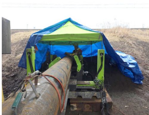
Shown above, some of the site constraints of the Portal North Bridge Project. NJ based trenchless contractor Kmetz Inc utilized their HHB equipment on this project and now deploys it on nearly every project where rock is anticipated
