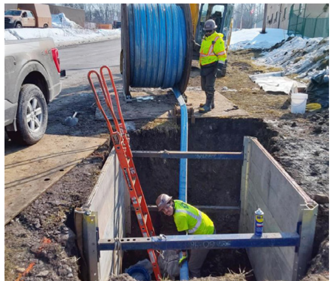
Quick installation eliminated the need for a temporary bypass during construction
