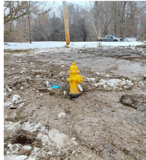
Another timely and successful critical rehabilitation completed
