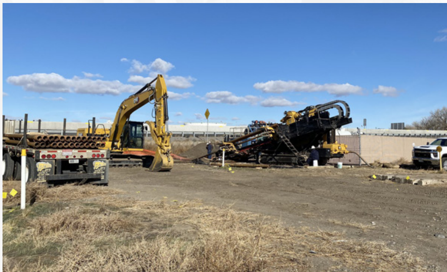
Drill rig set up at HDD entry
