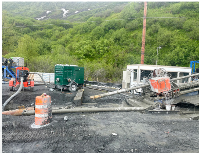
Nearly the entire alignment was completed by HDD, reducing surface impacts
