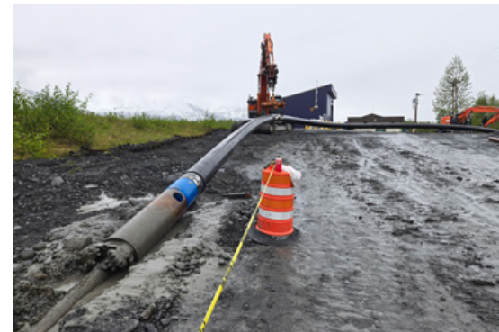
Drills were redesigned for longer lengths with deeper profiles to mitigate IR risk
