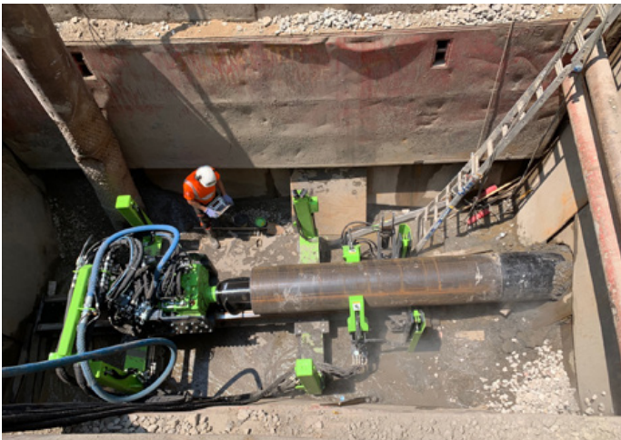
Figure 4. The Drill machine shown in the launch pit. Rotation is provided by hydraulic pressures and compressed air fed through the rotary unit to the auger to operate the hammer. The technician holds the remote with live display to monitor and adjust all drilling parameters
