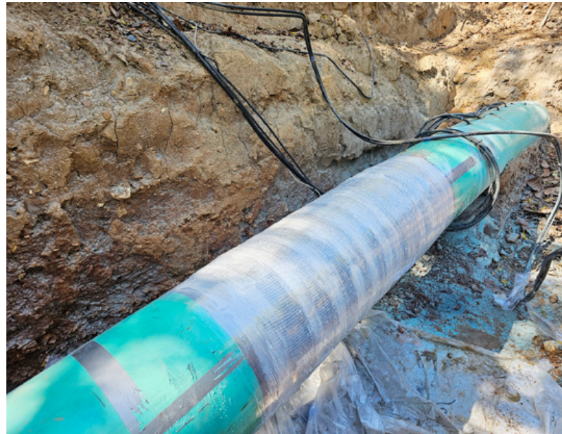
Denso's Composite Pipe Repair Systems are advanced, non-metallic solutions engineered to restore and reinforce the structural integrity of pipelines affected by corrosion, wall loss, or mechanical damage—without the need for welding or shutdowns
