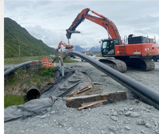
Ballasting with water was required for pullbacks exceeding 1,000 feet
