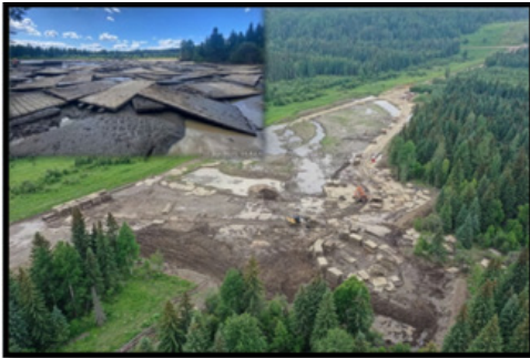
Figure 10 - Entry Pad Flooding
