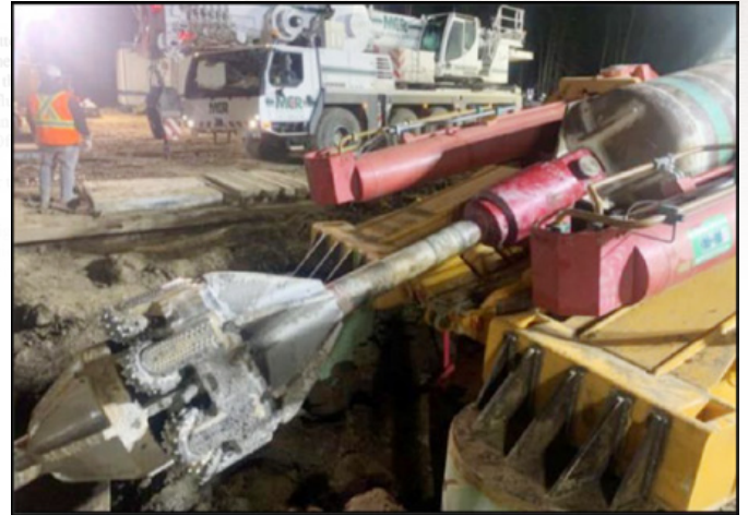
Figure 20 – Product Pipe Installation Successful
