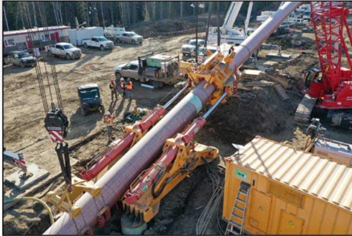
Figure 19 – Thruster used during Pullback
