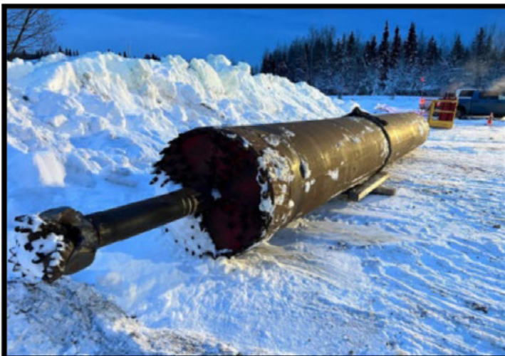
Figure 6 – Forward boring Unit
